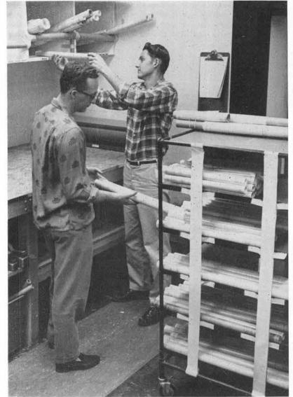
MICROFILMING PROCESS BEGINS for engineering drawings when William Lewis, foreground, and Ralph Lovvorn check in tracings and sort them numerically by size. Approximately 380 tracings are logged in each day for processing by the Section.
